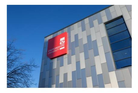
Aluminium rainscreen cladding systems are lightweight, durable, cost-effective, offer a wide range of colour choices, are suitable for both new build and refurbishment schemes, and have a design life in excess of 40 years. Ash & Lacy offers a 25-year system warranty utilising high-quality engineered products and finishes, to give our customers confidence in our ability to deliver long-lasting system solutions.
