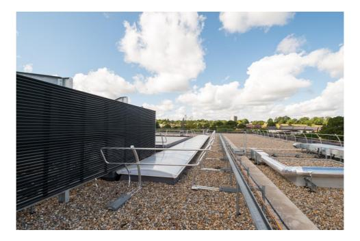
A combination of nine Marvault rooflight systems and four Mardome glass domes were installed at Ark Kings Academy in King's Norton, Birmimgham. This combination of rooflights and glass domes allowed natural daylight to be admitted into areas where vertical light, through windows would not reach.
