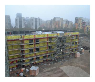
Unlike internal air barriers, which can be complex and costly to install due to the need to accommodate building services such as electrical, lighting, heating and drainage systems, positioning an air barrier on the outside of the insulation simplifies the process of maintaining the envelope's integrity, as there are less building services and structural penetrations to be sealed.
