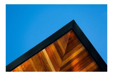
Around 100 linear metres of the bespoke profile was fitted to the sloping surface, vertically and horizontally, coming together with specially-made compound corners which join the profiles together at the change of direction. Pressed from heavy-gauge aluminium, the 625mm width coping was seven-times bent and the finished profile helped the couple to achieve their concept vision.
