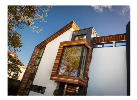
Guttercrest's aluminium fascia and coping can be polyester powder coated in a wide variety of RAL colours and textures, including stone effect finishes, ensuring their low maintenance and long life.
