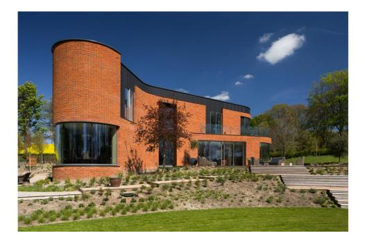
Guttercrest coping has a weather struck top, but can be made flat or dual pitched. As well as being low maintenance, they are lightweight, adaptable and easy to install. In addition to the coping system, Guttercrest also designed, manufactured and supplied bespoke faceted curved cill flashing for the window areas and drip flashing on parapet walls. Window flashings measured 3mm thick and 150mm width, while brick flashing measured 300mm width. The flashings are also available as true curves.
