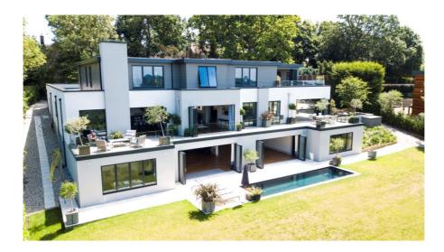
Complementary aluminium coping is used for the parapet/balcony walls of the property, providing a striking contrast to the white rendered walls. The wall copings are fabricated from marine grade aluminium at Guttercrest's Shropshire manufacturing facility. Unlike stone wall copings, these are lightweight, versatile, adaptable and very quick to install. They are also 100% recyclable, perfect for the eco conscious developer.
