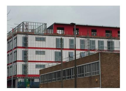
Wraptite, the only self-adhering vapour permeable air barrier certified by the BBA, combines the important properties of vapour permeability and airtightness in one self-adhering membrane. The introduction of Wraptite will make a significant contribution to the building's thermal performance by preventing lateral air movement.
