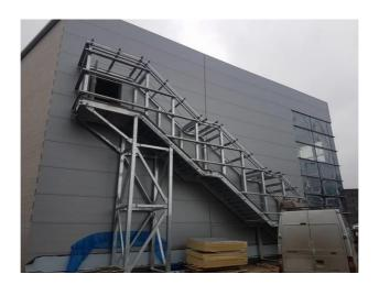
Guttercrest worked with installers GutterTec, to provide cladding which would house the steel-framed fire escape. Roof and vertical cladding were bespoke-pressed single skin to be fitted with hidden fixings and with minimal framework to keep the structure as lightweight and economical as possible.
