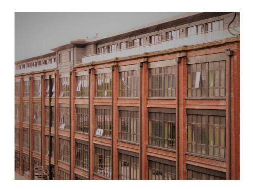
Guttercrest have supplied over 100 large cast rainwater hopper heads, each with personalised name plates and over 700 metres of aluminium downpipes to the £60 million redevelopment of the old Cadbury factory site in Keynsham, Bristol.
