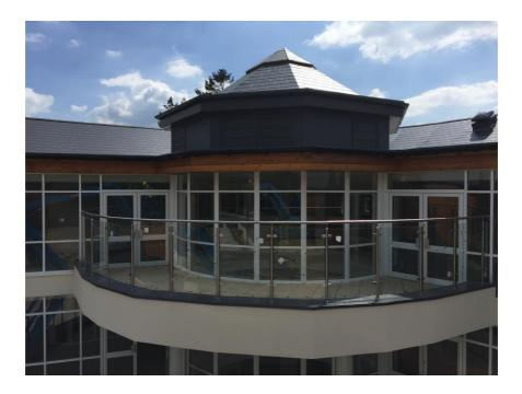
Rainwater goods including half round gutters and round pipes, fascias and soffits were supplied and fitted to the turreted area of the care home.
