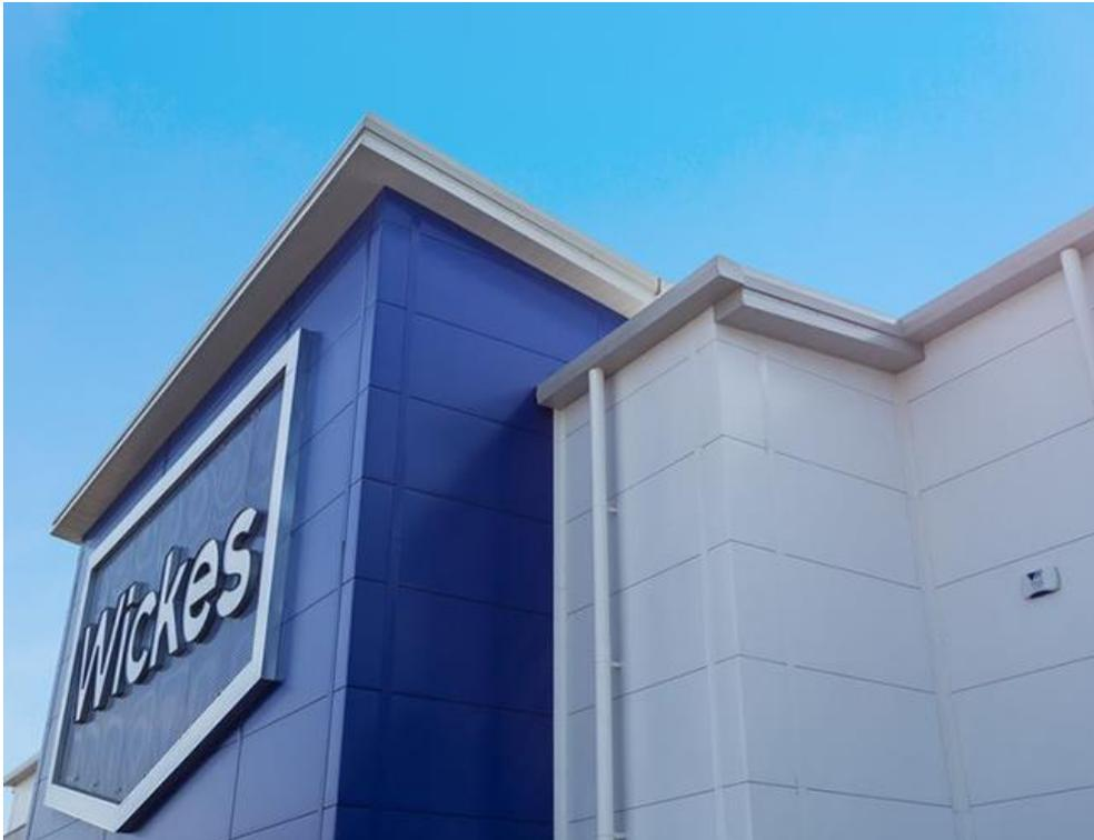
Guaranteed system performance and sustainability were key drivers in selecting the pre-finished steel cladding for the new, steel-framed Wickes store at Cirencester. The client, Travis Perkins, specified Tata Steel branded products to meet the design and performance criteria.
