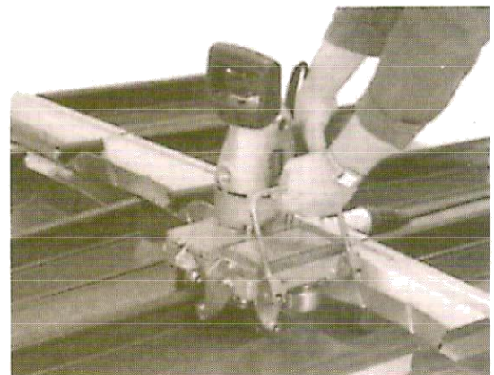
MECHANICALLY SEAMED LAP
