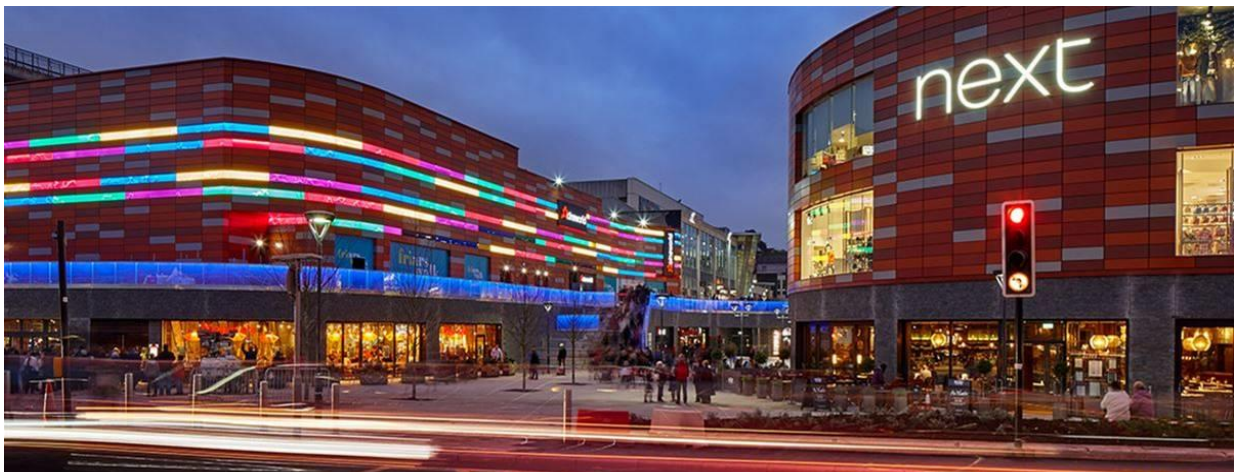
Friars Walk Shopping Centre, Newport, Gwent
