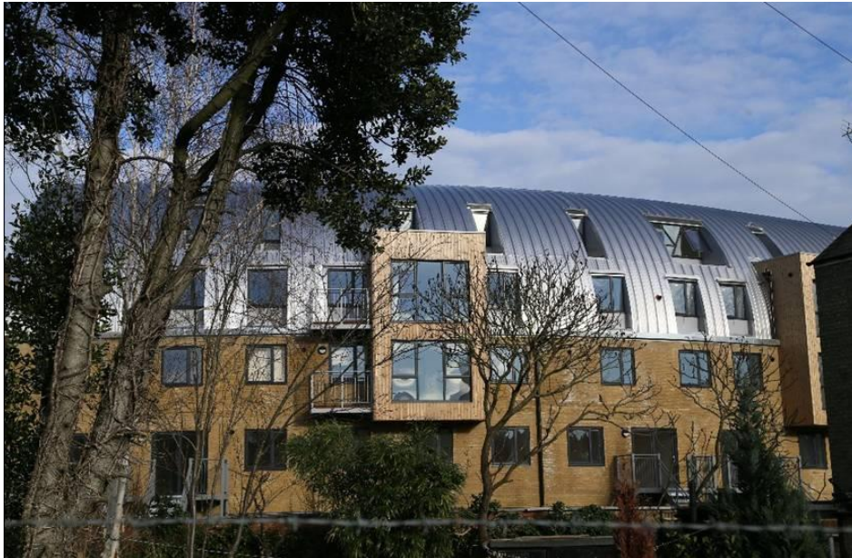
Residential development, Marshgate Drive Hertfordshire
