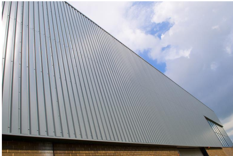
Deeside Leisure Centre, Cheshire. Image courtesy of Tata Steel
