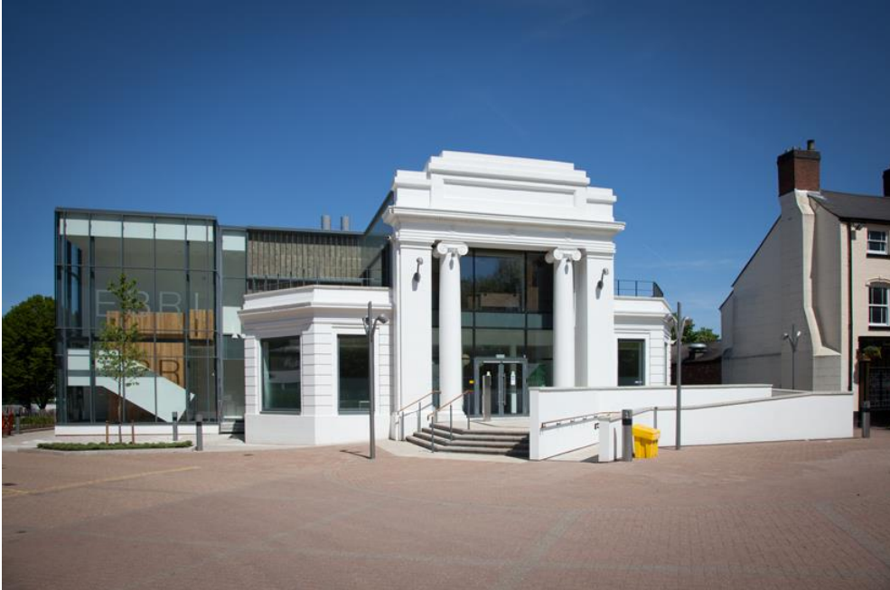
The EBRI building at Aston University. Image © Tim Cornbill
