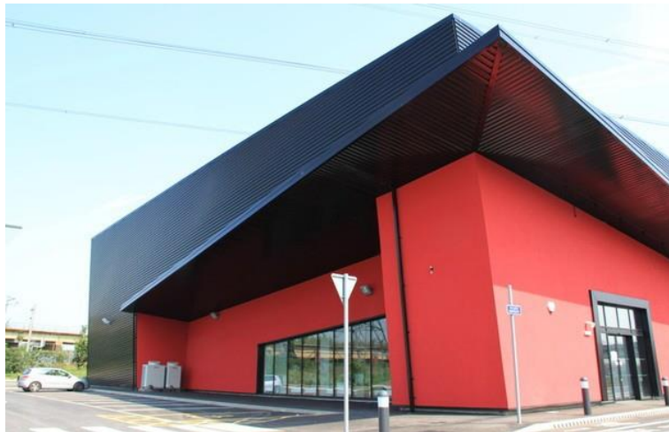
Crossrail Training Academy, Ilford east London Image courtesy of CA Building Group
