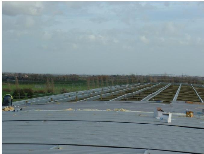
*Image 1: Undulating/out of position purlin*
