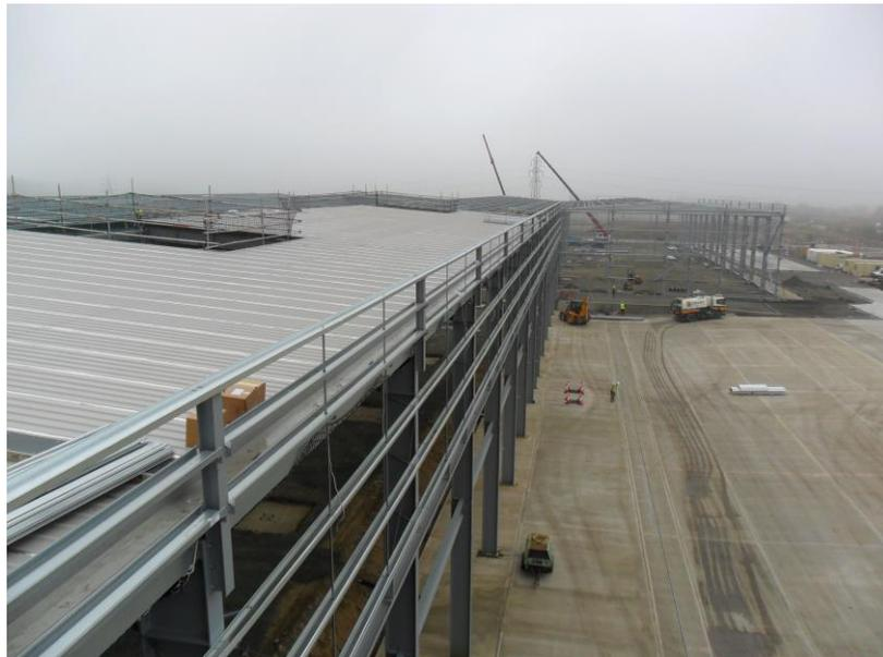
*Image 4: Primary and secondary steelwork properly installed*
