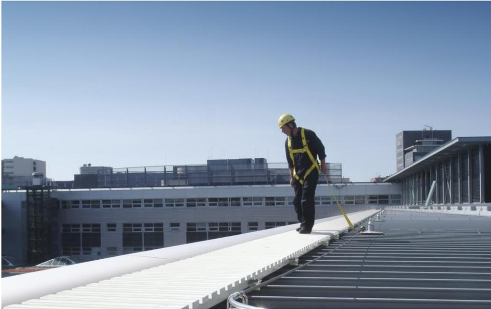
*Collective fall protection of guardrail and walkway with accompanying cable system providing access to restricted areas. Image courtesy of Latchways plc*
