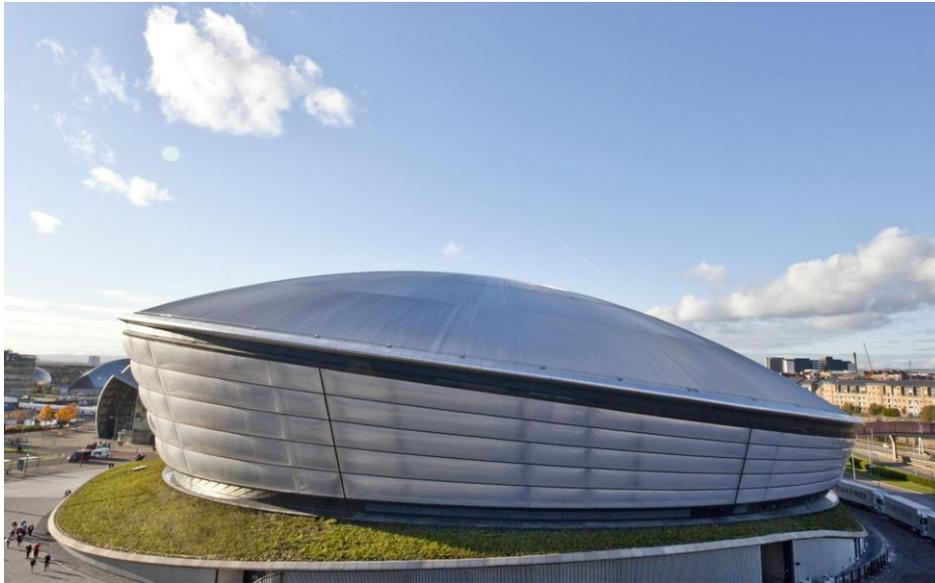
To meet the performance criteria specified by Foster + Partners, the resulting multi-layer acoustic Kalzip roof build-up achieves a U-value of  $0.20 \text{ W/m}^2\text{K}$ , a weighted Sound Reduction Index of 53 decibels and a sound absorption performance of Class A.
