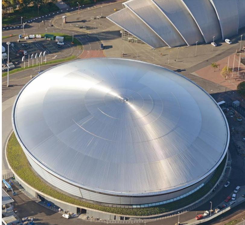
Kalzip's aluminium standing seam system with a weighted Sound Reduction Index (SRI) figure of 53 decibels was specified by Foster + Partners for the 125 metre span roof of The SSE Hydro in Glasgow. This impressive, imaginatively designed and flexible 13,000 capacity live entertainment venue was built for the Scottish Exhibition Centre Ltd by Lend Lease and the shallow domed Kalzip roof was installed by Martifer UK.
