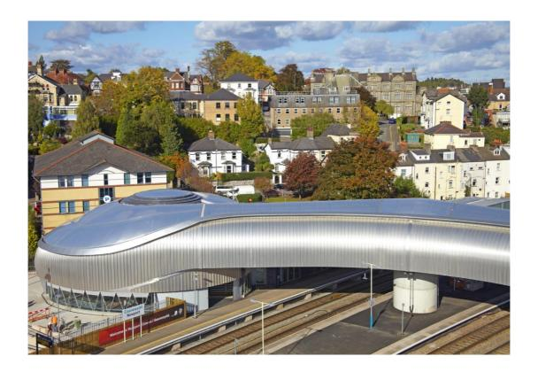
Over 1,000 individual Kalzip aluminium standing seam sheets have been installed on Network Rail's stunningly designed new station at Newport, South Wales. As well as straight, tapered and smooth curved Kalzip sheets, many revolutionary Kalzip XT profile sheets of various shapes and sizes were used for significant parts of the link footbridge and concourse buildings where the aluminium cladding is curved both on plan and in section.
