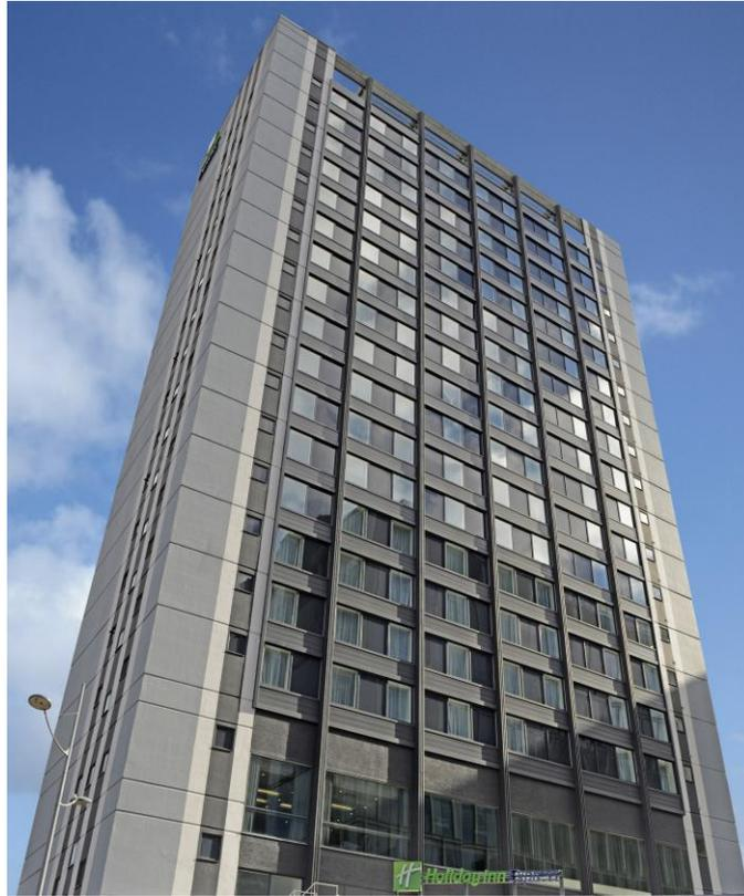
Over 600 square metres of Kalzip's quick-fit FC rainscreen system panels have been used to help transform the façade of a 72 metre high, tired-looking 1970s office block into an impressive new 224 room Holiday Inn Express in Snow Hill, Birmingham. Falconer Chester Hall (Liverpool) was the architect and the low cost Kalzip FC rainscreen panels were recommended and installed by the experienced curtain wall and window contractor, Continental Installations Ltd.
