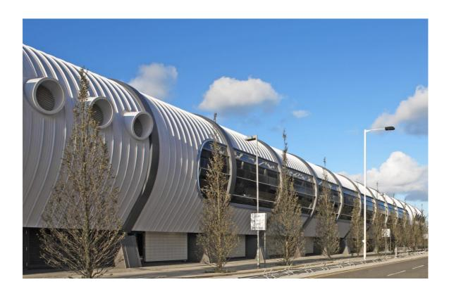
Over 6,000 square metres of Kalzip aluminium standing seam sheets, a similar quantity of Kalzip aluminium structural decking and an impressive array of Kalzip fabrications (all materials PVF² / PPC colour coated to Matt Lilac 59BB63/066) were specified by Red Box Architecture for Sunderland City Council's striking new £20 million Sunderland Aquatic Centre. Built by Balfour Beatty Construction, the long, flattened tubular shaped aquatic centre houses NE England's largest and Olympic-sized pool.
