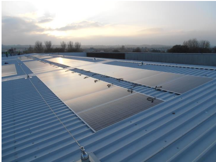
PV installation in progress on Deeside Leisure Centre
