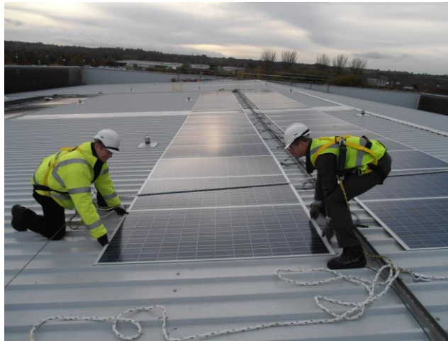
Lightweight Solon PV module bonded onto a Trisomet roof panel
