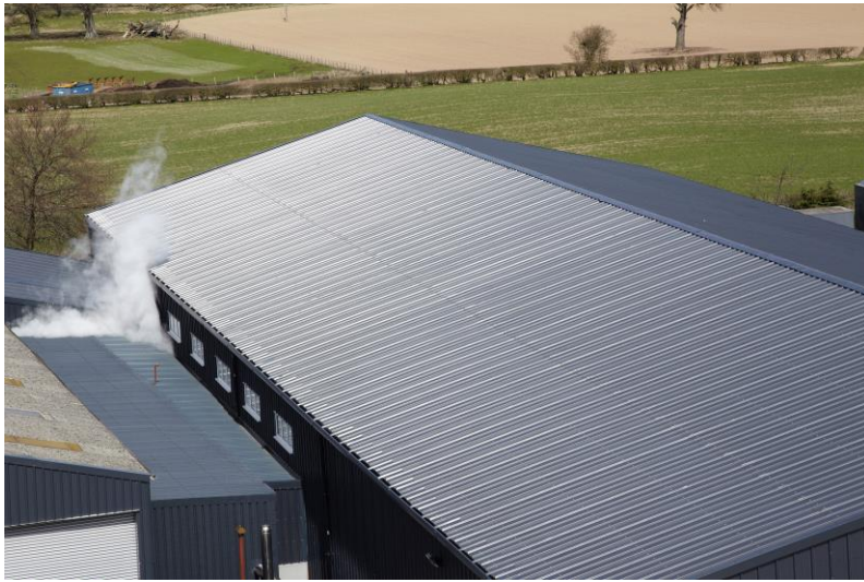
Insulated roof panels at Radnor Hills Mineral Water Company, Powys Courtesy of A Steadman & Son
