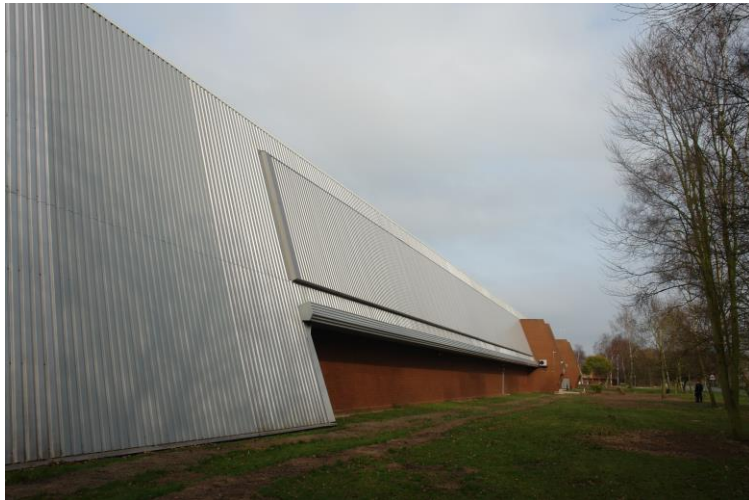
SolarWall was used at Jaguar/Land Rover at Leamington Spa
