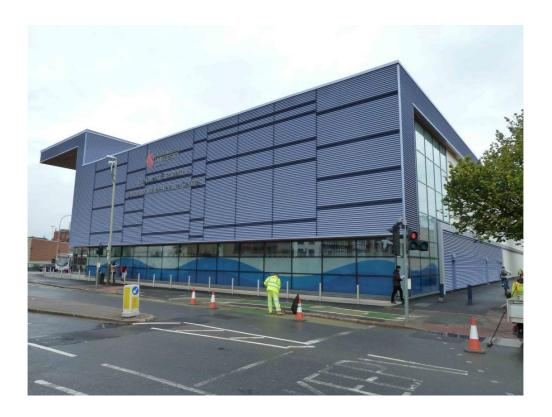
The new Queen Elizabeth II Diamond Jubilee Leisure Centre at De Montfort University in Leicester is a master class in the use of louvres to create a stunning building design. Designed by S&P Architects, the roll formed louvre profile and live louvre cladding is part of the metal profile portfolio of Architectural Profiles Limited of Woodley near Reading.
