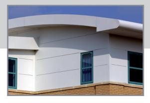
These are used to provide the end detail to a curved roof. The range of applications is extremely wide however, the curved fabrication invariably makes a strong aesthetic statement.
