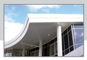
Fascias are used on vertical faces and soffits for the underside of horizontal faces. These items are often treated as cladding, however they are mentioned here because they are often used to create architectural features to complement or contrast with the main cladding system.
