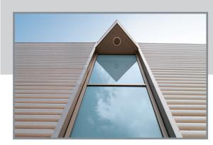
Window surrounds manage the interface between cladding and window frames. They can be used for purely functional purposes but can also provide a striking visual feature.
