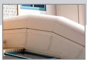
In this example, circular curved fabrications are used to create a rounded feature on a building; they are often used on the eaves.
