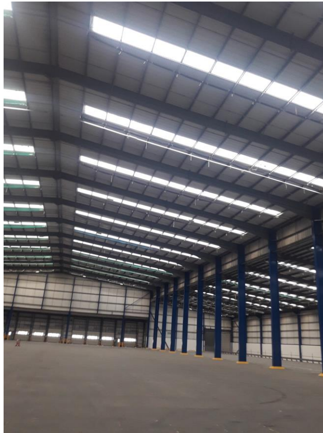
Rooflight replacement internal
