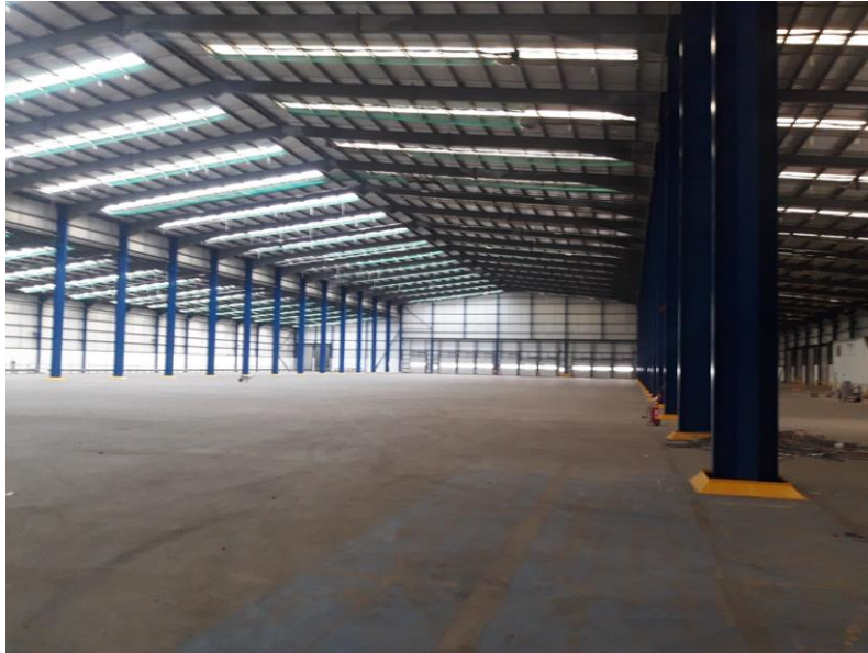
Zenon rooflights installed to the left hand slope
