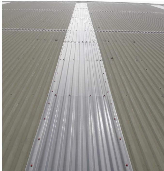
Rooflight replacement complete
