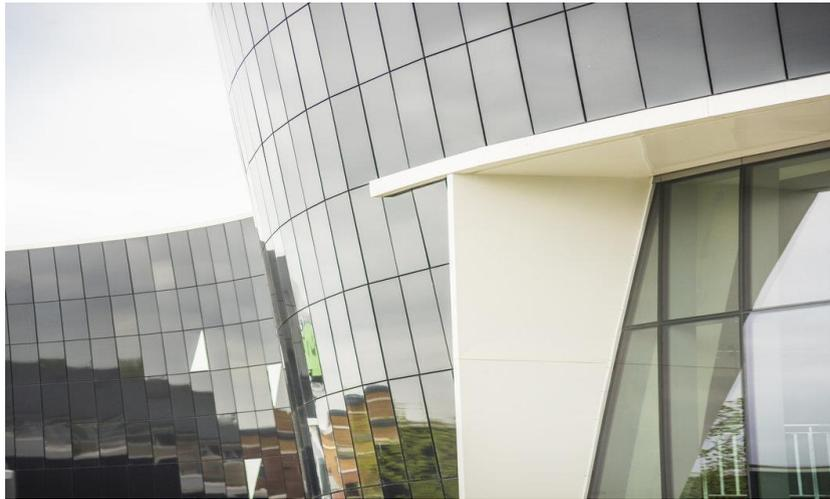
The Eurobond composite panel was specified in Colorcoat Prisma® pre-finished steel in White as the ideal inner skin of the building. This specification helped towards removing the second façade installation from the critical path and achieving weathertightness early on in the building programme.
