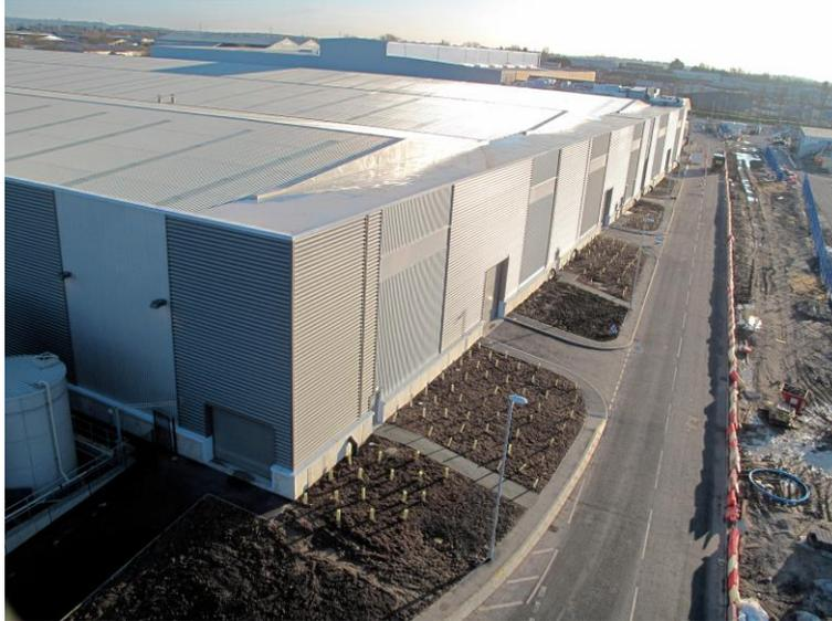
Tovi Eco Park Residual Waste Treatment Facility was built to provide mechanical and biological treatment of up to 417,000 tonnes of municipal residual waste annually. The facility includes three bio-stabilisation halls with large roofing spans and high imposed loadings – calling for a high-strength roofing product. The corrosive internal environment of the halls meant a super durable material was needed.
