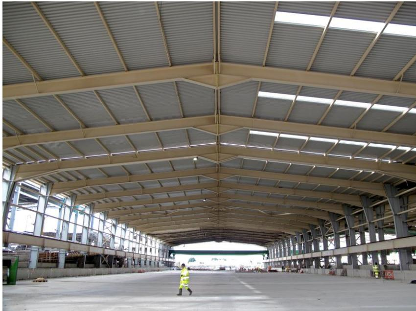
The size of the halls dictated a roofing solution with substantial spanning capacity. In addition, the shape and height (13.30m at ridge) of the hall roofs, combined with the openness of the site, meant that the roofs needed to withstand high imposed loading (snow drift loads up to 4kN/m<sup>2</sup> and wind suction up to 1.98kN/m<sup>2</sup>). The live load was 1.5kN/m<sup>2</sup>. Close overlapping of the roof deck was required for weather sealing whilst also accommodating roof lights.
