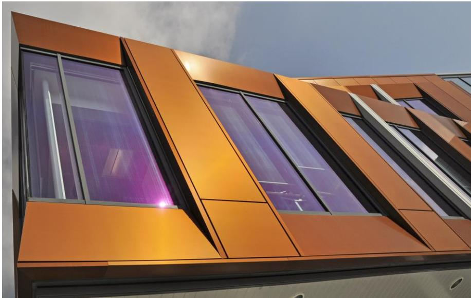
The new 60,000 square feet building features both Sotech's Secret Fix FC attachment system and their Through Fix Cassette (TFC) rainscreen system. Sotech explains, "The Sotech Optima FC system was selected for the project due to the precise coordination between panel and substructure that presents a pristine appearance without the use of visible fixings. The TFC rainscreen system was also selected as accurate installation is both simple and speedy."
