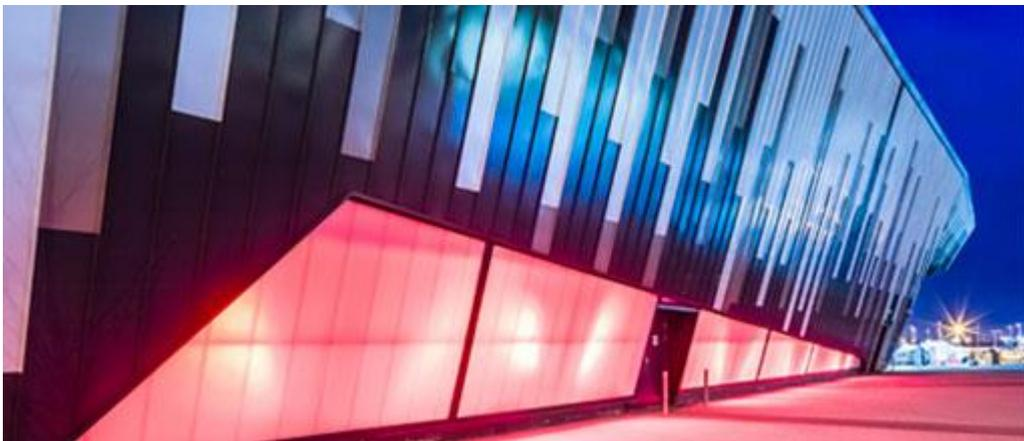
A lightweight polycarbonate panel, Marlon Clickfix1040 system has integral interlocking connections that simply click into place forming glazed areas of unlimited size and shape. The 40mm structured polycarbonate glazing panel has 10 insulating walls to achieve a U-value of 0.99 W/m<sup>2</sup>K, for a high performing and thermally-efficient glazing solution.
