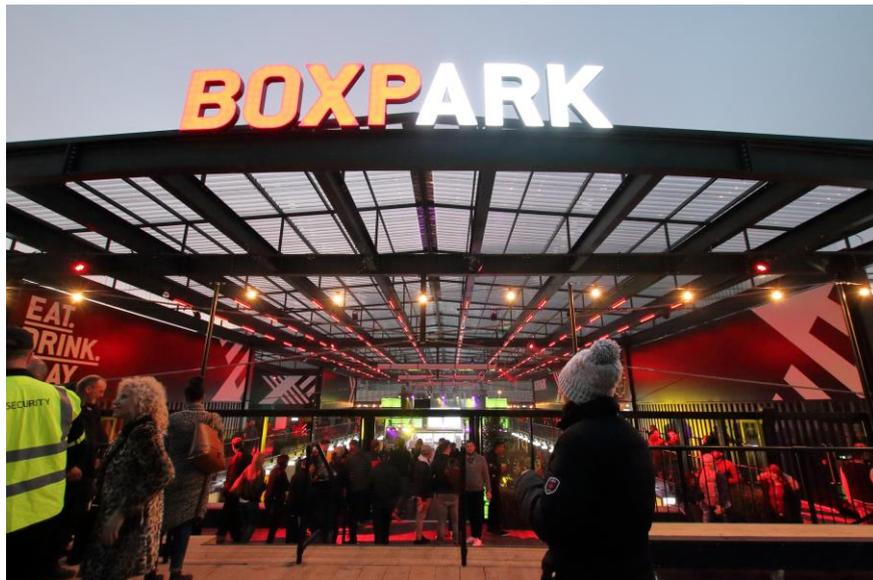
Commenting on the project, Daniel Isaac, area business manager at Brett Martin Daylight Systems said; “We recommended a pitch of 5 degrees to avoid any water ingress issues in the space below and advised on fixing methods which included 2mm thick EPDM dry seal compression tape at the end laps due to longer overlaps.”
