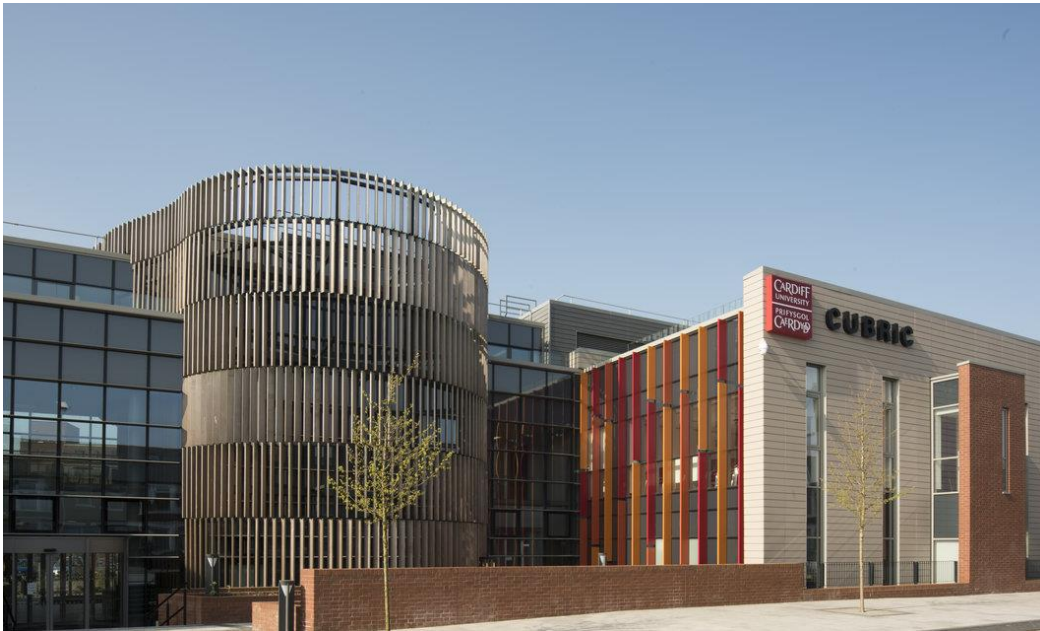
CUBRIC Centre, Cardiff. Image courtesy of Eurobond Laminates
