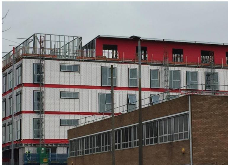
Wraptite, the only self-adhering vapour permeable air barrier certified by the BBA, combines the important properties of vapour permeability and airtightness in one self-adhering membrane. The introduction of Wraptite will make a significant contribution to the building's thermal performance by preventing lateral air movement.
