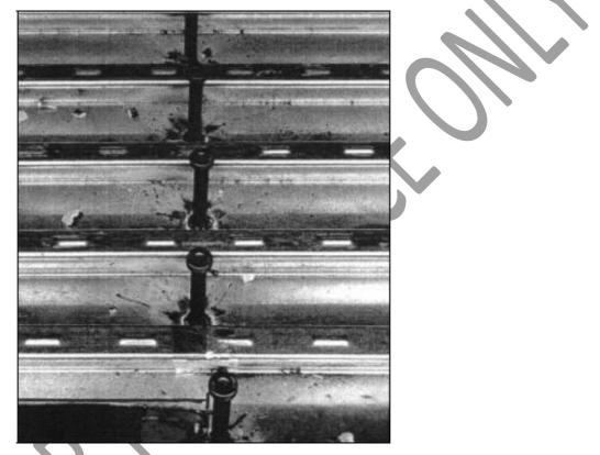
Figure 5.7 A typical run of stud shear connectors
