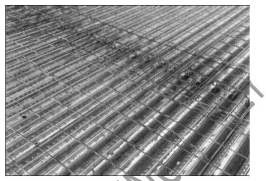
Figure 6.3 Decking and fabric reinforcement – ready for casting the concrete
