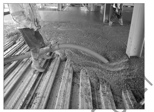
Figure 6.4 Pumping of fibre-reinforced concrete
