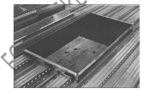
**Figure 4.12** A typical trimmed opening (immediately after deck laying, prior to fixing the edge protection and reinforcement around the opening)
