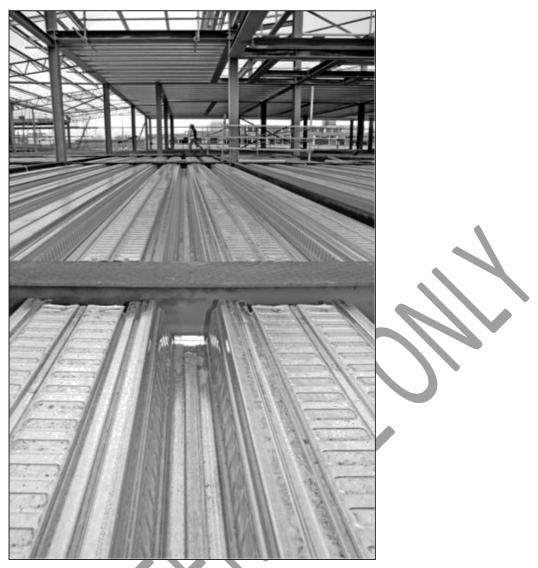
Figure 7.5 View of Slimflor construction using ComFlor 225 decking.
