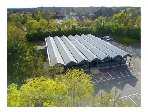
With a £125,000 investment, the refurbishment of Cypress House was completed in April 2017, with decorative exterior cladding and a high performance roof, both featuring non combustible insulation with inherent thermal and sound insulation.
