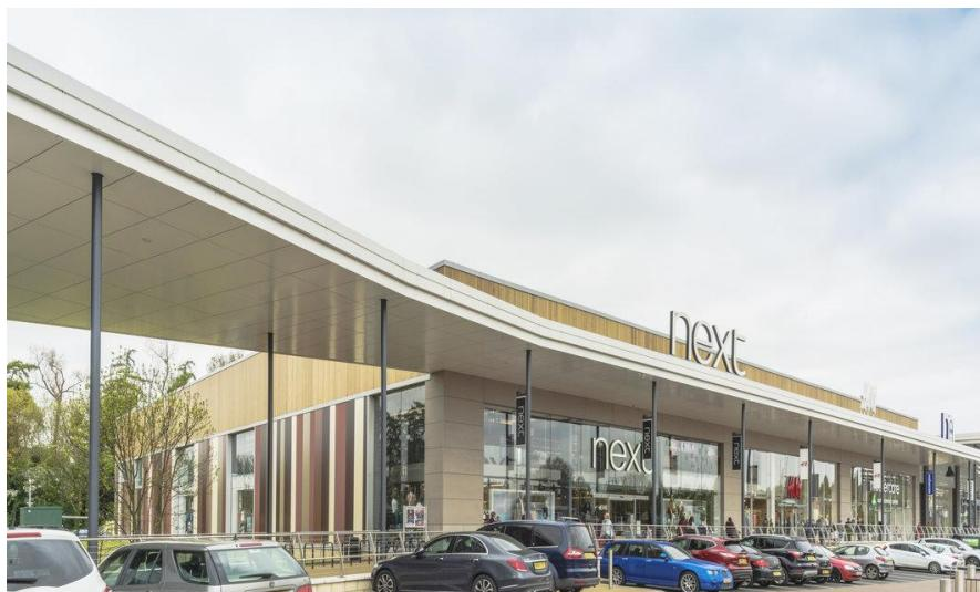
Europanel has been vertically installed on the sides of the buildings which utilises the secret fix joint, architectural flatness and 1mm modular flexibility creating a visually pleasing façade. From an aesthetic point of view, the Eurobond non-combustible panels are extremely flat and maximize the impact of the colour scheme.
