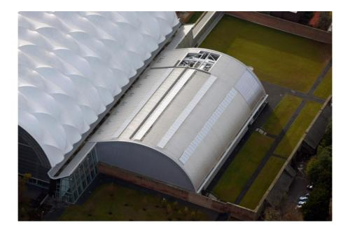
Highly versatile, Brett Martin's Ritchlight mono and dual pitched skylights can be produced in any run length so the design opportunities are endless. Ritchlight mono and dual pitched skylights offer a wide range of glazing options and U-values as low as 1.1 W/m<sup>2</sup>K, far exceeding the thermal requirements of Part L of The Building Regulations.
