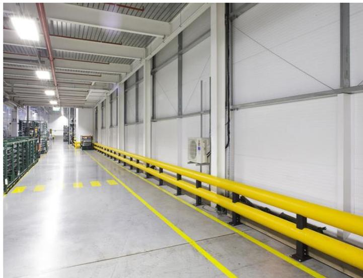
The cladding was installed by IRC Carocelle who constructed the extension's envelope using Tata Steel's high quality Trisomet® 60mm insulated panels for the wall and Trisomet® 80mm insulated panels for the roof.
