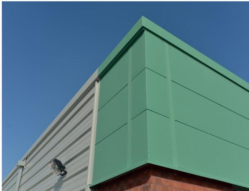
Tata Steel's technical department advised the architect that the Trisomet® 135 would be required to achieve a U-value of  $0.15\text{W}/\text{m}^2\text{K}$  on the roof while Trisomet® 120 and Trimapanel® would actually exceed the figure set for the wall – achieving U-values of  $0.16$  and  $0.17\text{W}/\text{m}^2\text{K}$  respectively. Guidance was also provided on issues such as the arrangement for dealing with rainwater run-off and the interfaces with sections of timber cladding.
