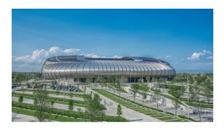
Members of Kalzip's design team in the UK were closely involved with creating the free-flowing geometry, finessing the design to simplify the fabrication and installation process; without compromising the architectural integrity. This included paying special attention to the hip areas and also designing the distinctive 'gills' which punctuate the aluminium envelope.
