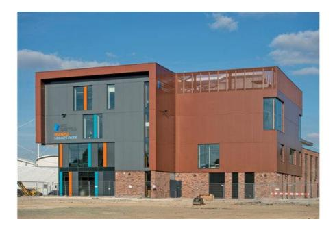
The final specification involved a single installation of Europanel manufactured from Colorcoat Prisma® by Tata Steel in Slate Grey and Helios (F5 Extra 200mm V Groove) and Rainspan (a composite panel providing structural support for rainscreen systems) to provide the combination of an impressive finish, completing the project in time and on budget.
