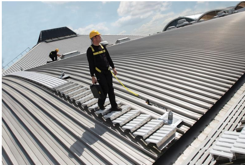
Cable system and walkway. Image courtesy of Latchways plc
