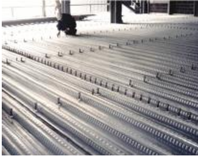
Profiled steel decking prior to concrete pour
