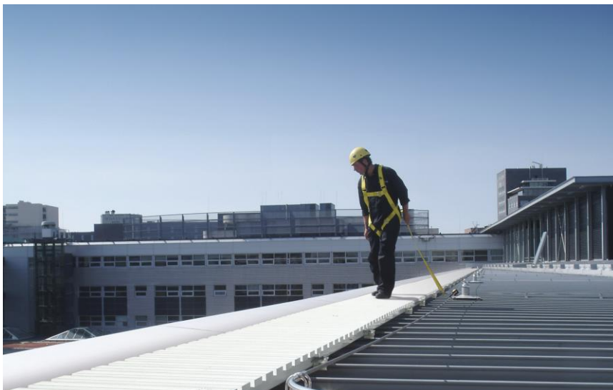
Cable system and walkway
