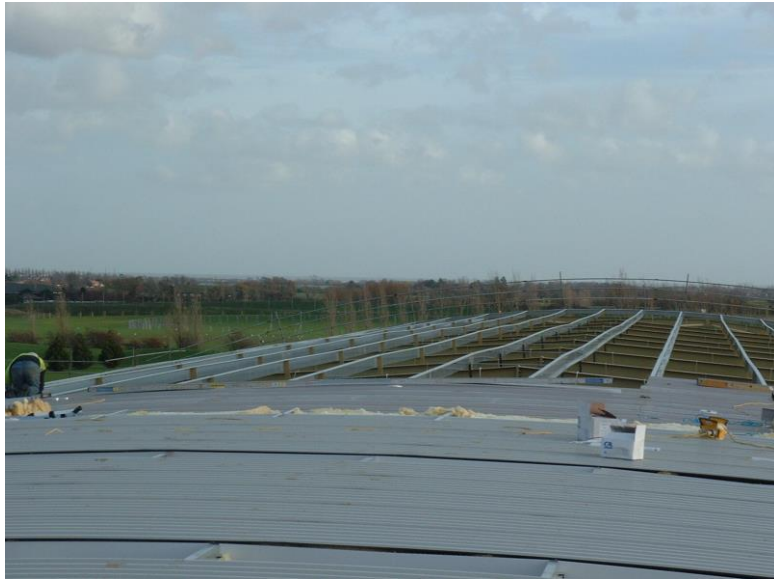
Image 1: Undulating/out of position purlin
