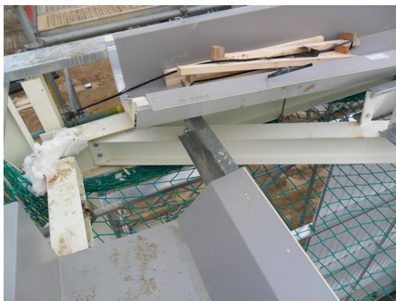
Image 4: Purlin/gutter clash
