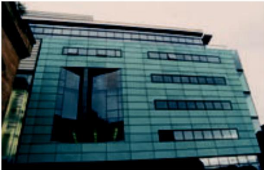
Modular panels and rainscreen
