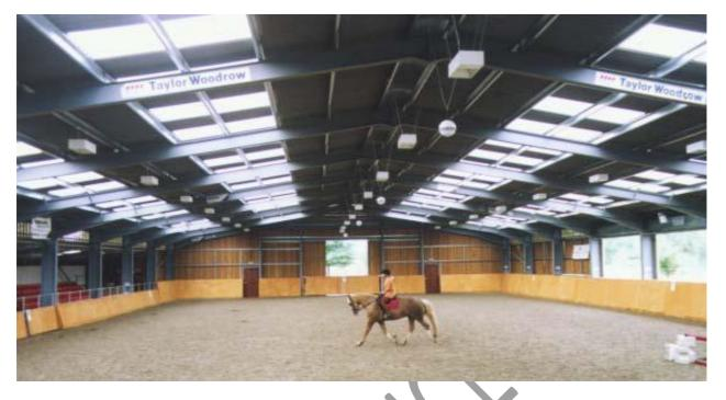
inclusion in future revisions to the Building Regulations, has predicted the daylight levels in the horizontal and vertical planes inside typical large span buildings (assuming even rooflight layout, without any significant obstructions) using the latest computer modelling techniques.
