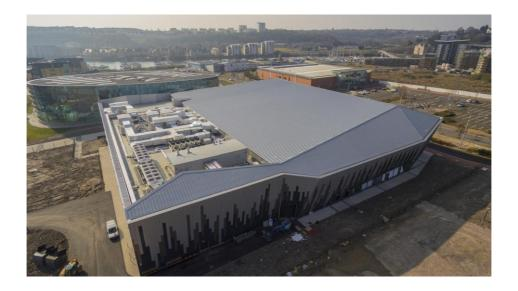
This unique product was developed within Euroclad's timescales, managing to meet the stringent project specifications, even with a variety of acoustic and thermal testing included as part of the product development. The resultant engineered roof and wall systems were enhanced versions of well-established Euroclad assemblies, which outperformed the acoustic requirement laid out by the design teams.
